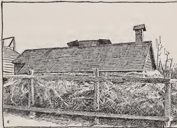
2737. An outside cellar, in which to store roots and tubers, and pots of resting stuff.
